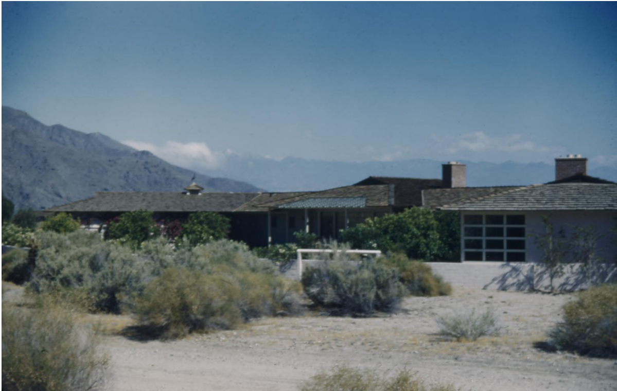
A 1974 image by Albert Frey of the rear elevation showing the multiple roof planes. Note the hitching post in the lower center.
