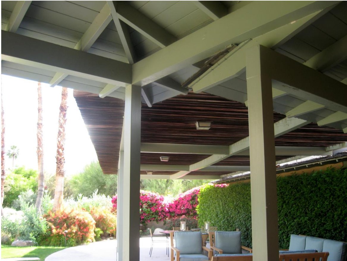
A view showing some of the intersecting eaves on the southern façade and Frey's 1968 redwood covered terrace addition. (Author photo. May 2019)
