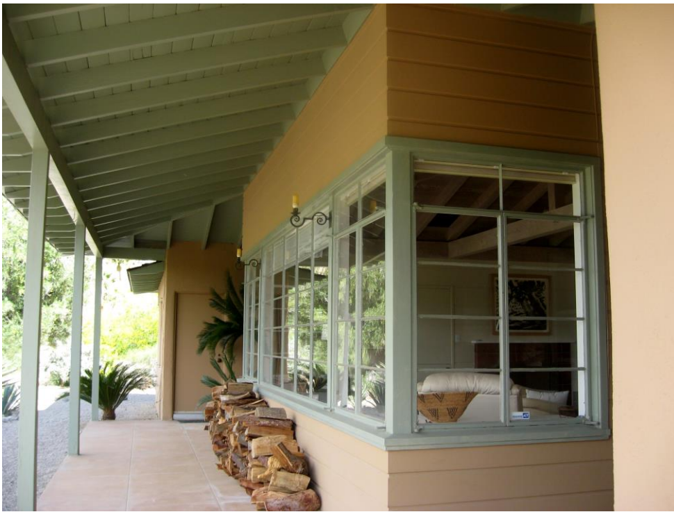
Looking eastward across front verandah. Note doorway to Frey's 1974 office addition. (Author Photo. May 2019)
