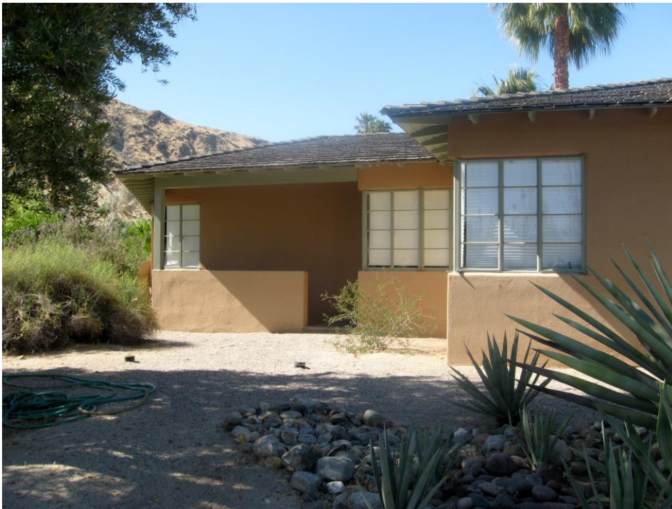
View showing opening to basement stairs. (Author Photo. May 2019)
